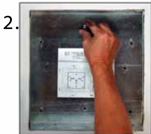
Insert COLUMBIA VORTEX® electrical box with provided fasteners.
