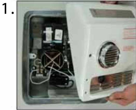
Remove your existing dryer. Leaving the existing electrical box in place.
