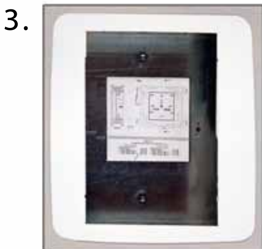
Mount Dryer flange onto the electrical mounting box.
